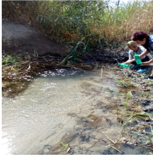
Photo 3.2 – Silted and overgrown with reeds collector K-1-2
