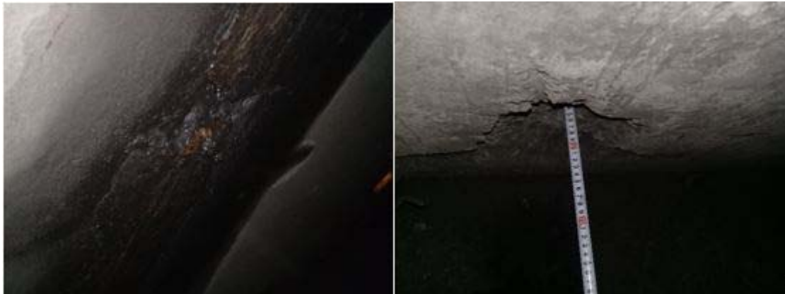
Figure 3.1 – Infiltration of water and leaching of the lining of the tunnel "Istiqlol"
