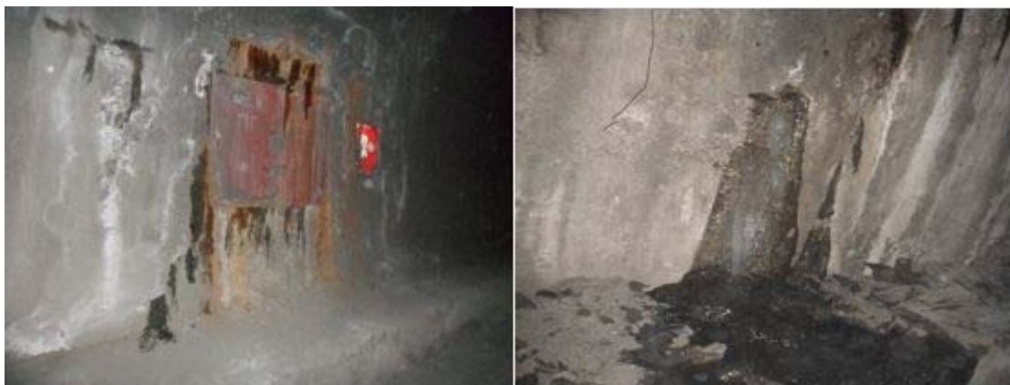
Figure 3.2 – Rust formation inside the tunnel and formation of ice on the lining of the tunnel "Istiqlol"
