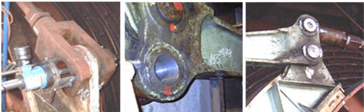
Figure 7 – Implementation of the method of repair and restoration of the hinged connection of the mechanism of the brake device of a mine hoisting machine
