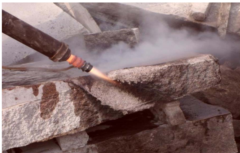
Figure 9 - A fragment of introduction into the torch flame to form steam/gas mixture
