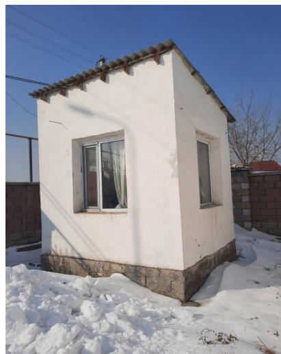
Figure 2. Greenhouse and cabin with MSW construction
