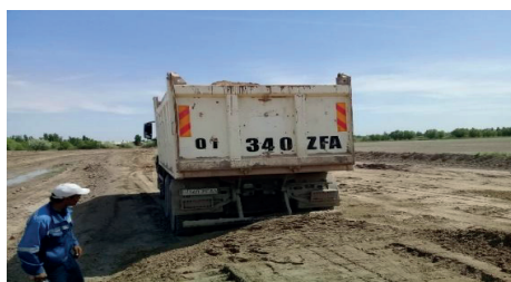
Figure 12. Delivery of soil by dump trucks
