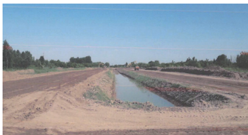
Figure 10. Excavation using an excavator and stacking soil along the channel.
