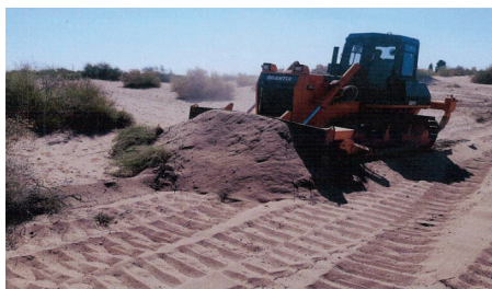
Figure 9. Bulldozer cutting through the vegetative layer
