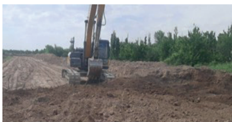
Figure 11. Leveling of the soil using an excavator
