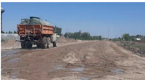
Figure 13. Moistening the soil to the optimum moisture level (machines and manually)
