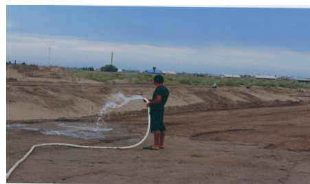
Figure 13. Moistening the soil to the optimum moisture level (machines and manually)
