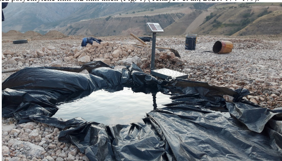
Figure 1 – Determination of the density by the “pit-hole” method of the first layer after two passes with a smooth roller with a vibrator turned on
